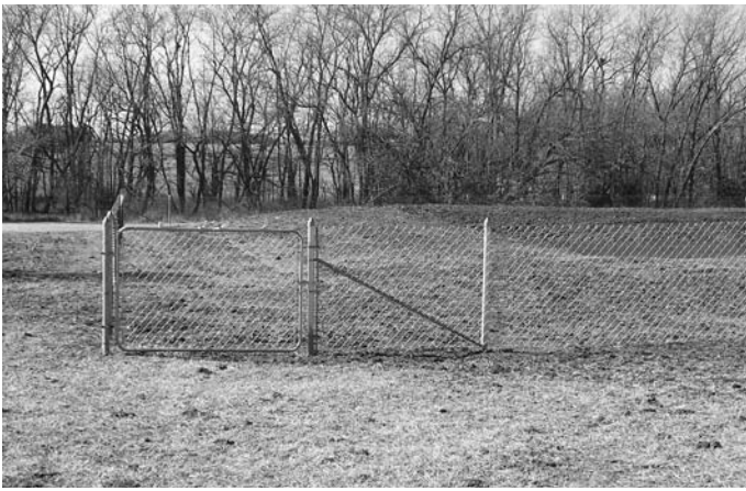
Figure 1. A lagoon with a good fence and gate outside the toe of the embankment.
